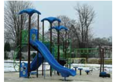
Carmelo Felix tot lot during installation work in January 2024
