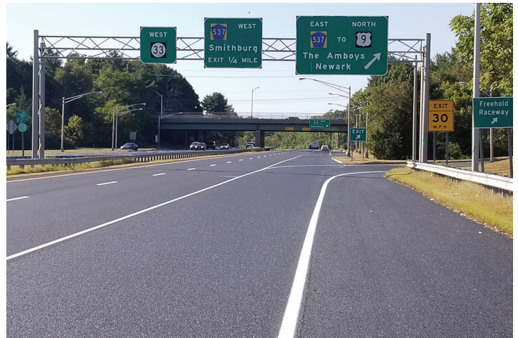
Pictured: Completed Route 33, CR 527 to Howell Road Pavement Preservation Project in Monmouth County.
